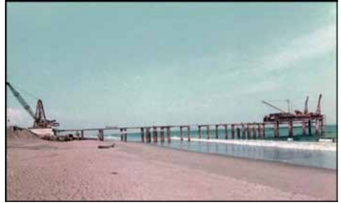
Figure 8. Marine bored piles in open sea condition
