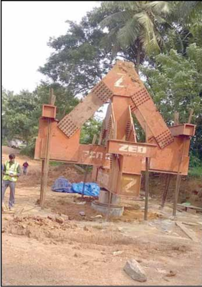
Figure 17. Pile load test using rock anchors
