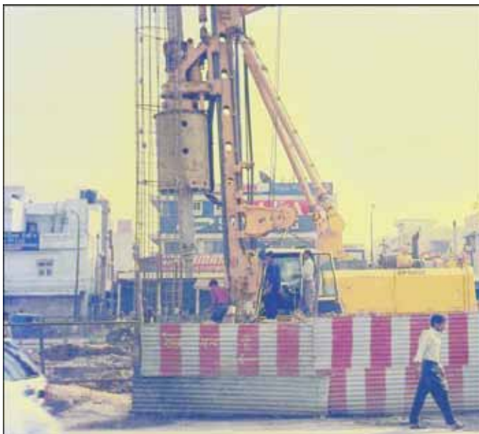
Figure 7. Bored piles under installation by Hydraulic Rig.
