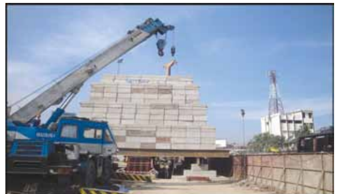
Figure 16. Pile load test using concrete blocks on loading platform
