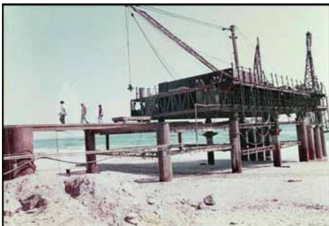
Figure 9. Mobile piling gantry.
