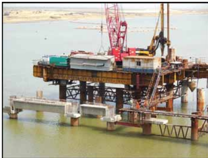
Figure 15. Hydraulic Rig mounted on mobile gantry
