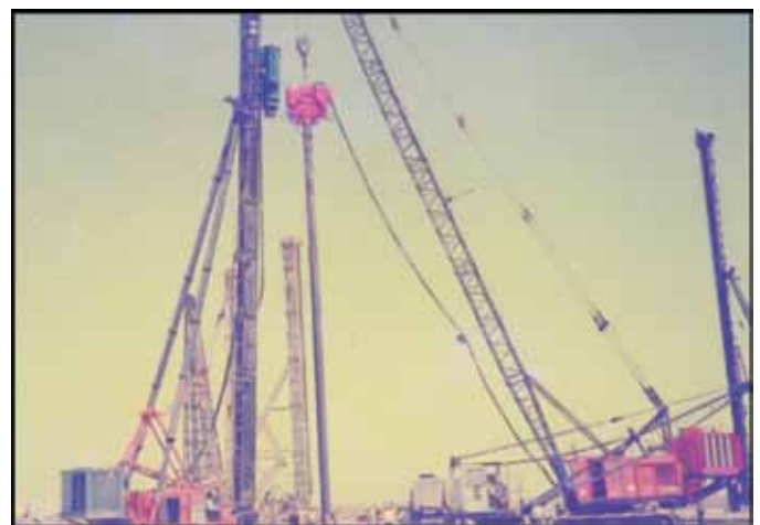
Figure 3. Pile Driver with Hydraulic Hammer and Vibrator-cum-Extractor on crane.
