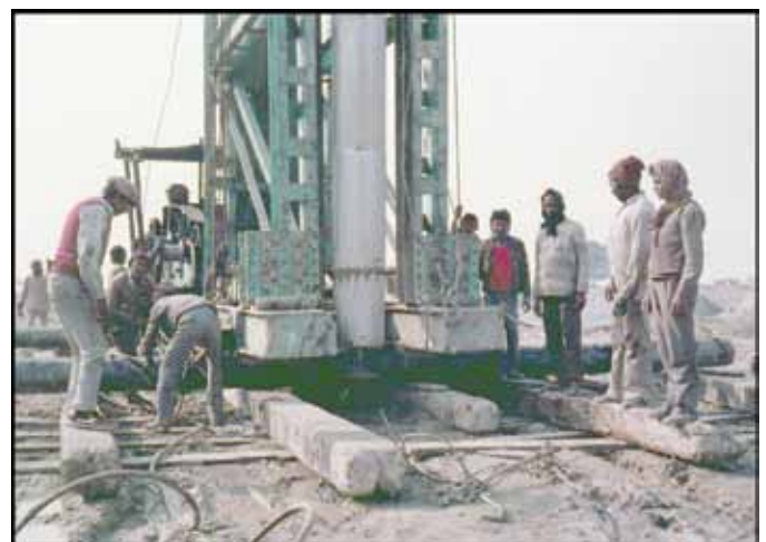
Figure 2. Conventional A-frame rig moving on roller over timbers.
