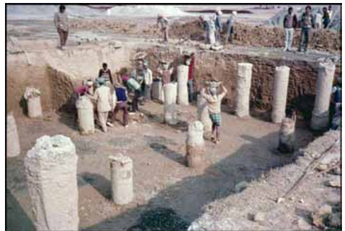
Figure 6. Sound pile concrete at pile cut-off level.
