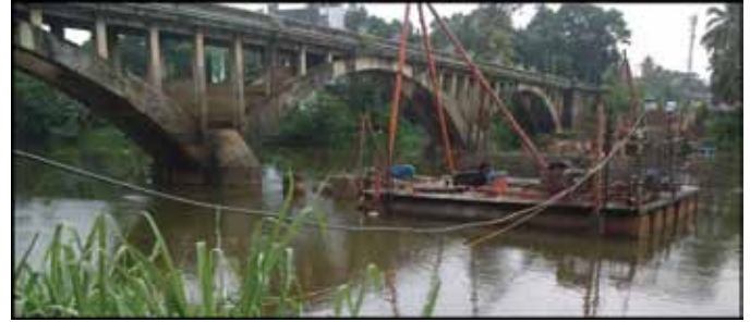
Figure 10. Bored piling using tripod rig
