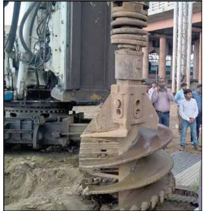
Figure 11. Rock Auger fitted to Hydraulic Rig
