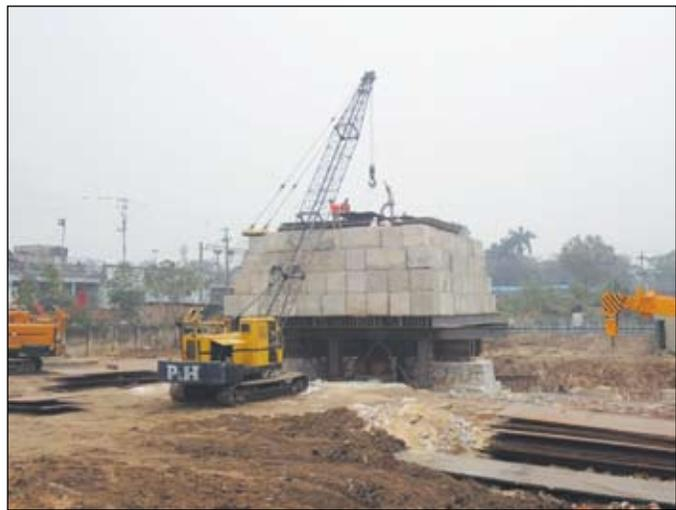
Figure 1. Kentledge being erected for load test
