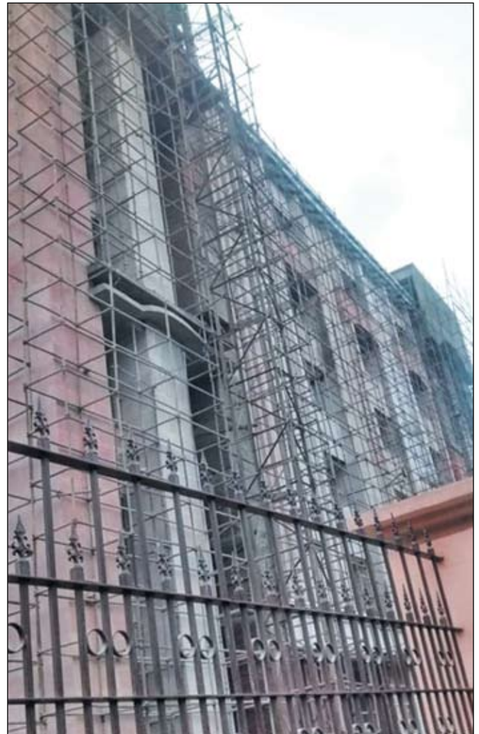
Figure 1. Scaffolding at a construction site
