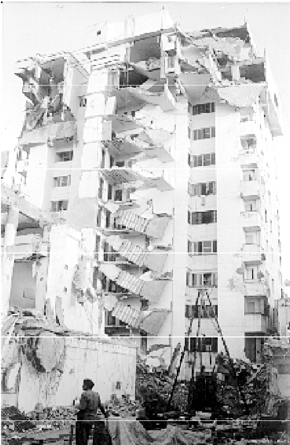
Collapse of a multi-storeyed building. Besides many reasons for failure, the main reason was additions and alterations done without considering earthquake forces
