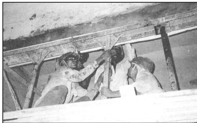
Figure 4. Propping the repaired beam
