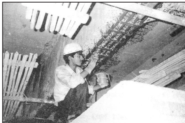
Figure 2. Application of protective coating on steel
