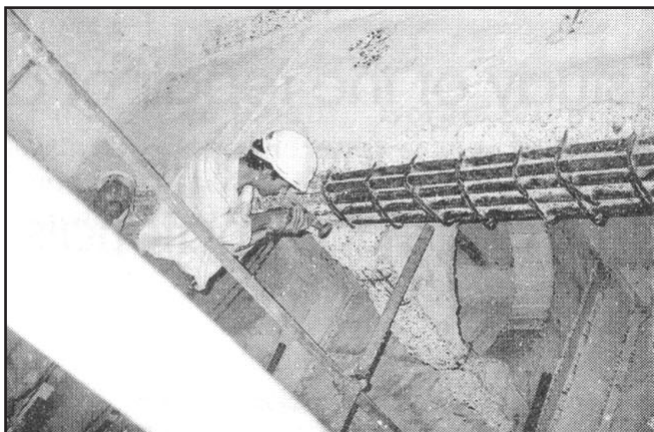
Figure 1. Cleaning corroded bars by mechanical wire-brush
