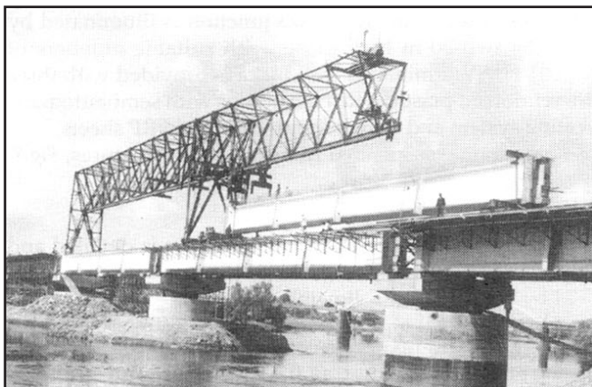
Figure 5. Launching of precast girders
