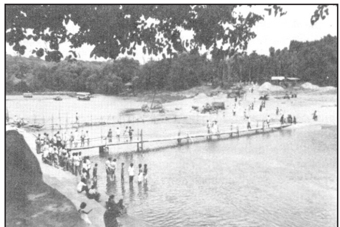
Figure 1. Temporary crossing at Sringeri prior to the construction of the bridge
