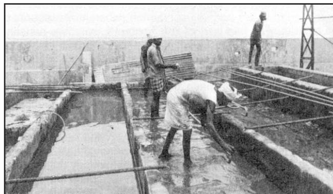
Figure 23. Protective coating to reinforcement
