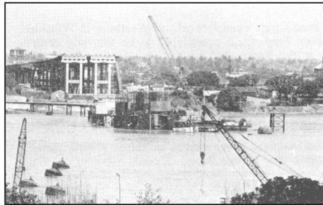
Figure 4. Upstream side floating caisson for foundation No. 3
