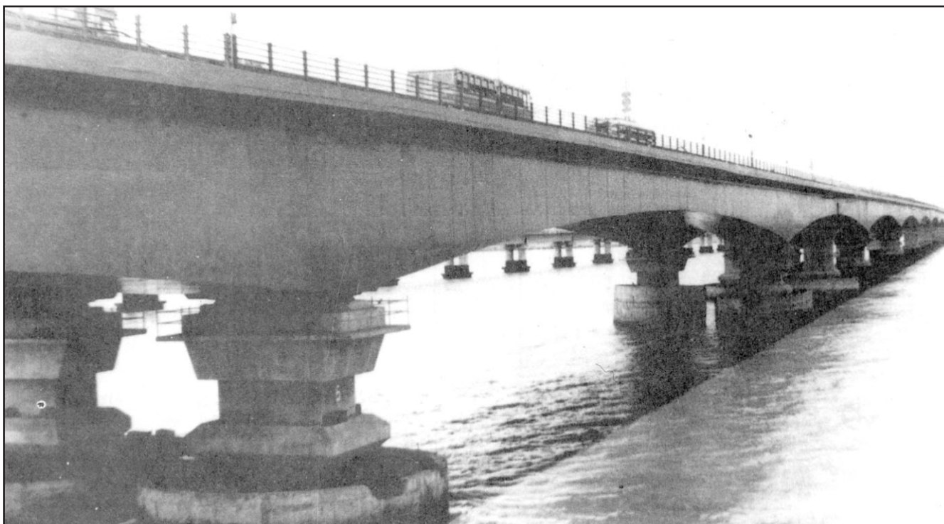
Figure 4. A view of the completed Thane Creek bridge
