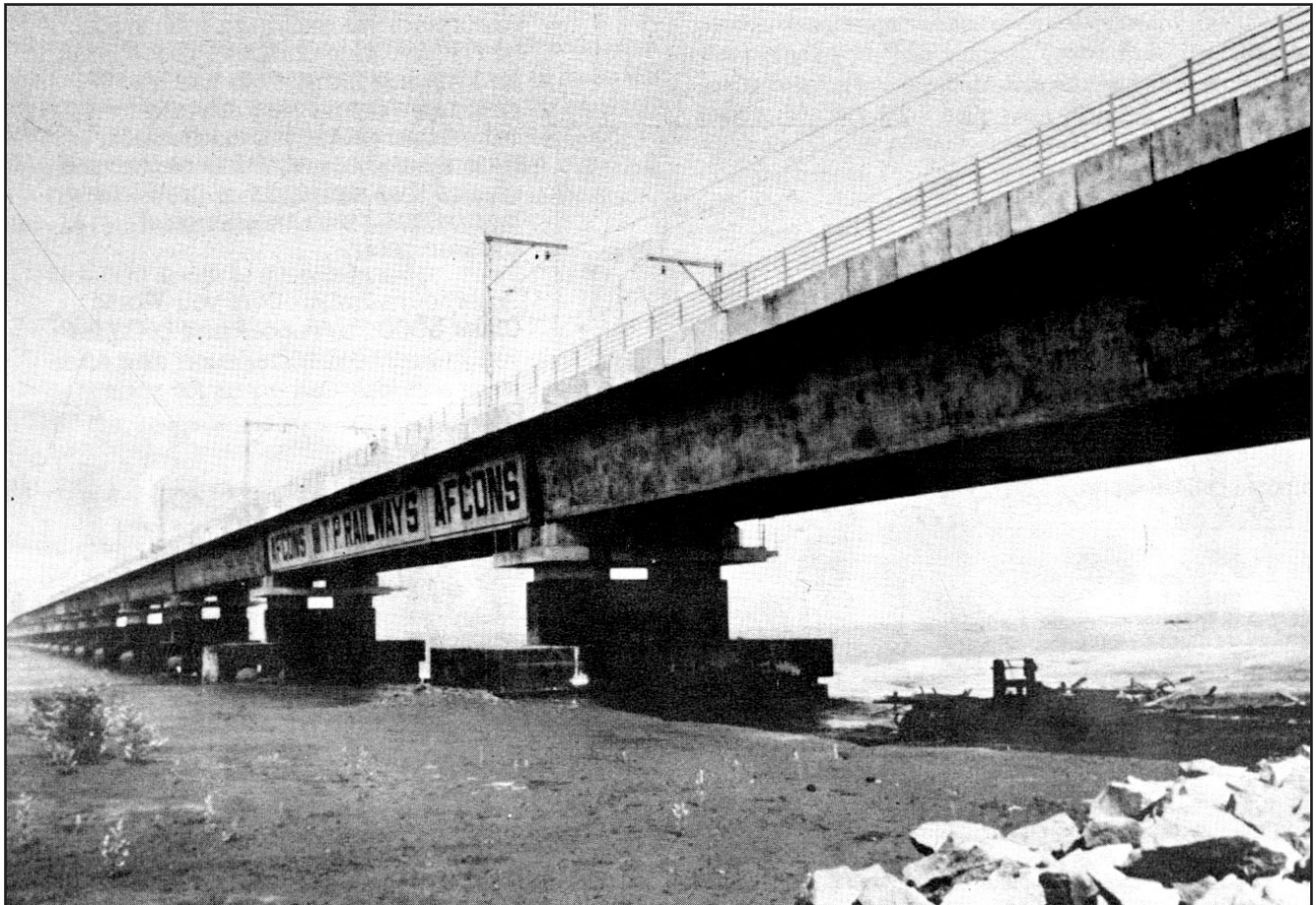
Figure 5. A panoramic view of the completed Thane Creek railway bridge
