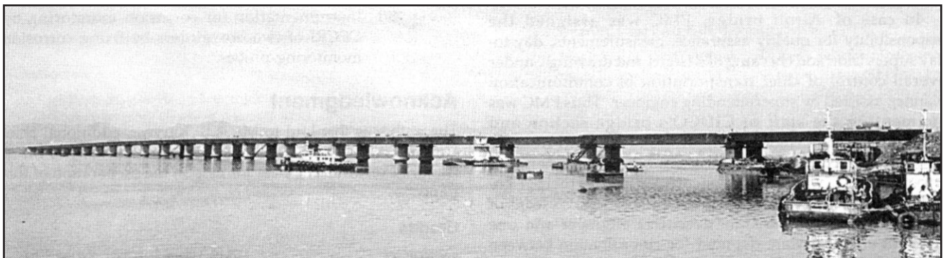
Figure 5. A view of the bridge nearing completion
