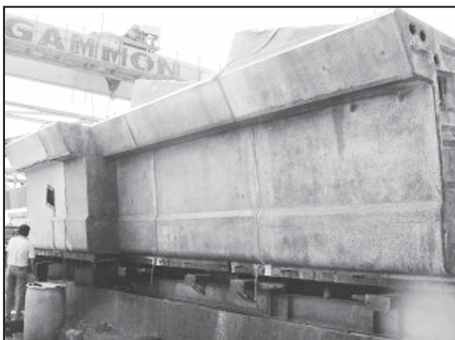
Figure 12. Precast segments on a long line
