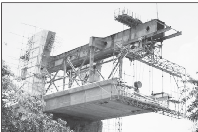
Figure 15. Start of cantilever construction
