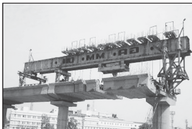
Figure 13. Lateral spans erection
