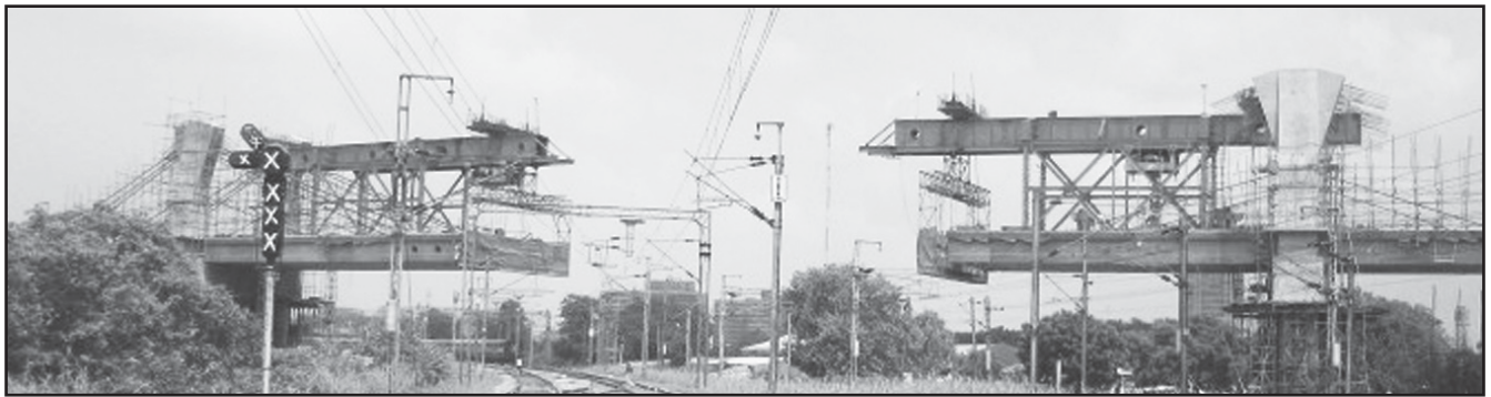
Figure 14. Cantilever construction of main span
