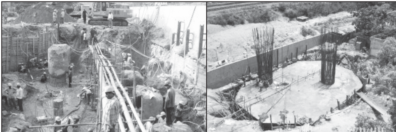
Figure 11. Works on pylon's foundations
