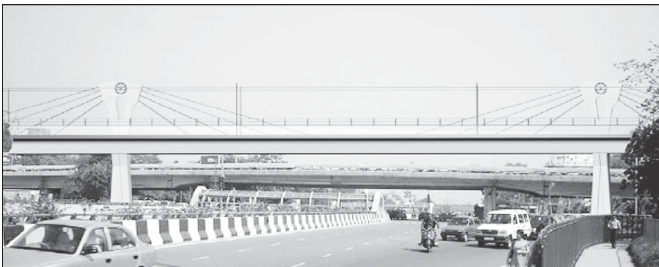
Figure 26. The Moolchand extradosed bridge
