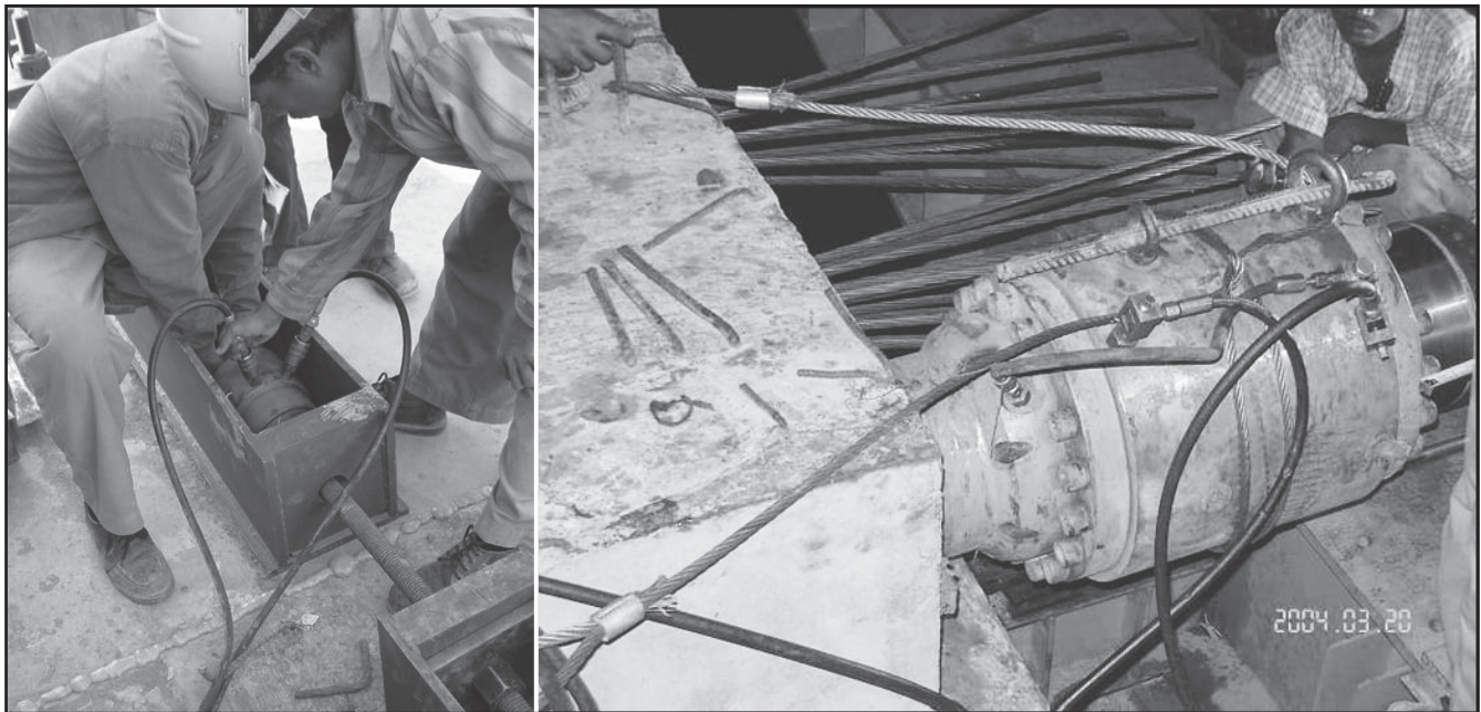
Figure 3. (left) Temporary prestressing operation (Right) final prestressing
