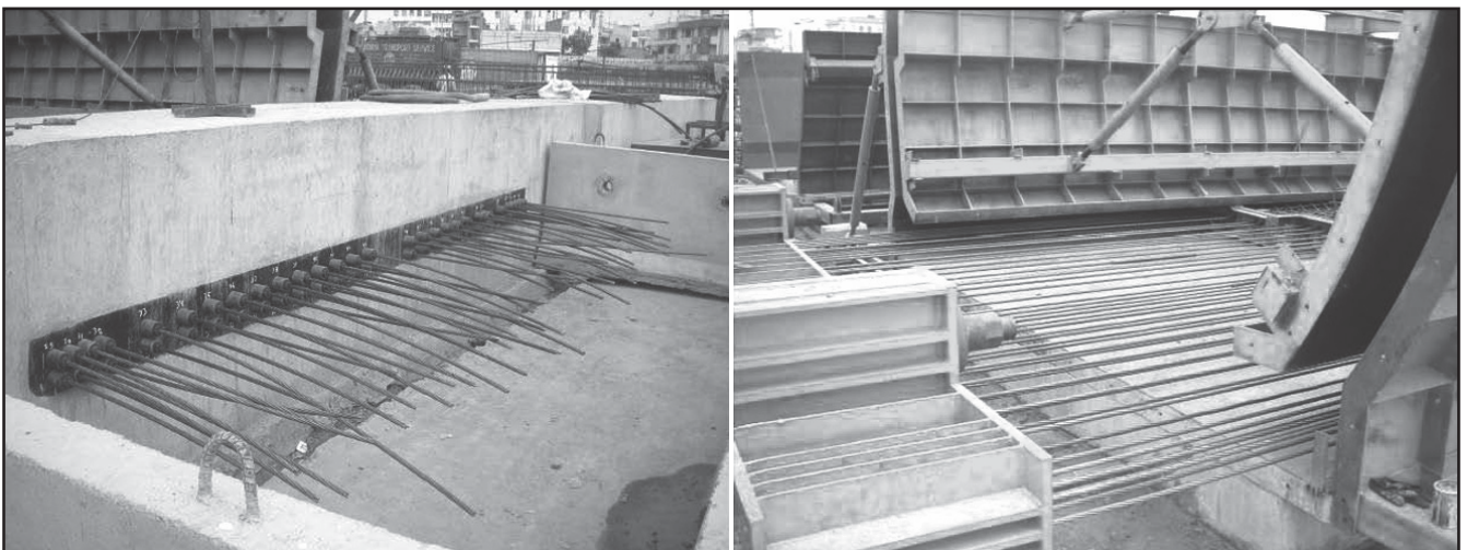
Figure 8. (Left) Prestressing passive end (Right) Prestressing active end
