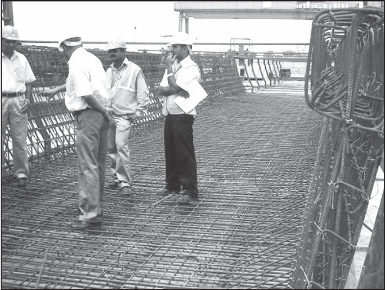
Figure 7. Rebar cage
