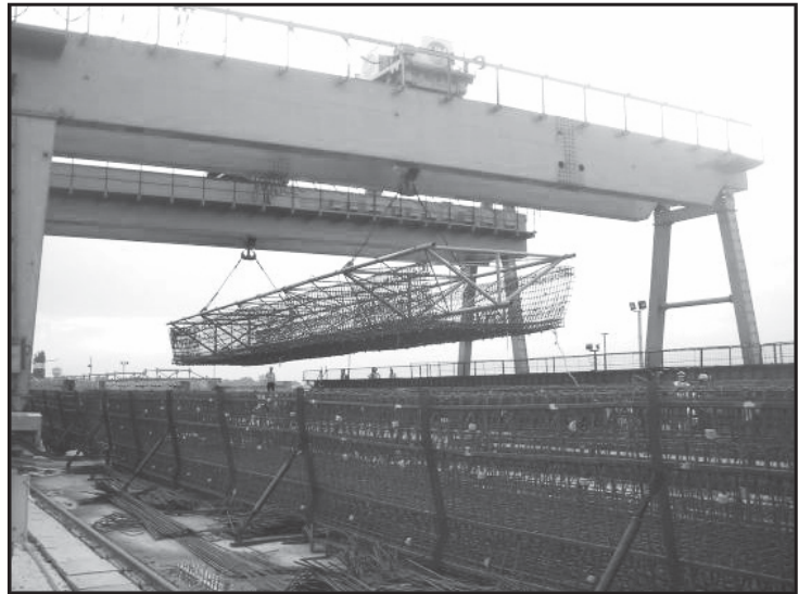
Figure 10. Lifting of rebar cage
