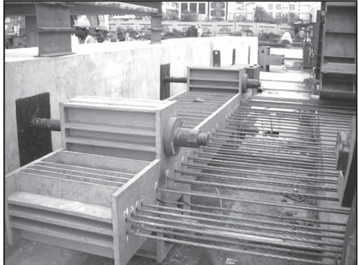
Figure 9. Pulling beam at active end
