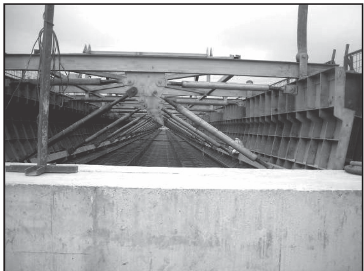
Figure 11. View of inner shutter after installation
