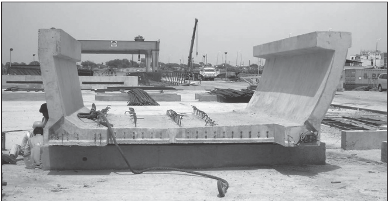
Figure 4. View of the precast U-girder on airport link viaduct
