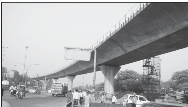
Figure 18. View of continuous span
