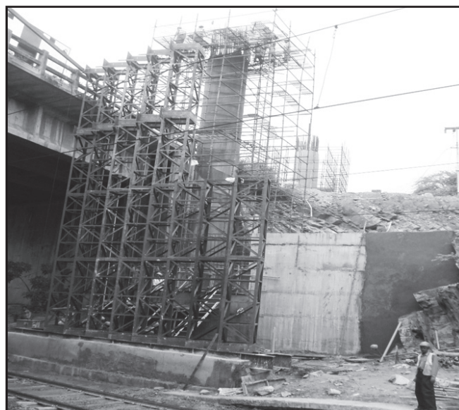
Figure 15. Foundation with counter weight near ROB
