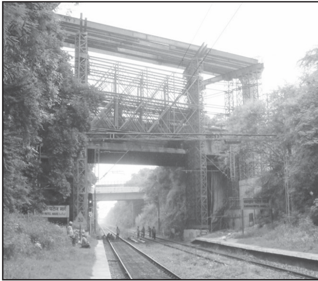
Figure 16. Temporary structure over railway line
