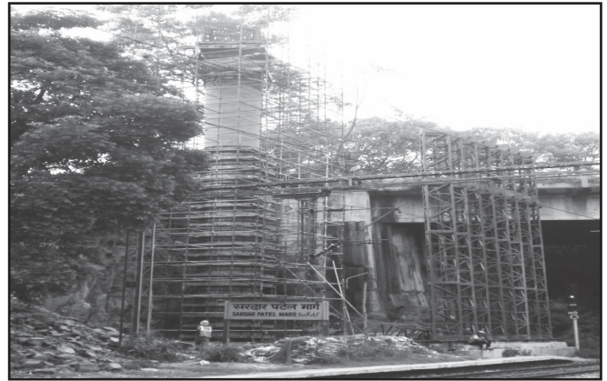
Figure 17. Highest pier, 20 m height
