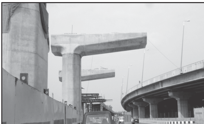
Figure 5. Cast in situ cantilever pier
