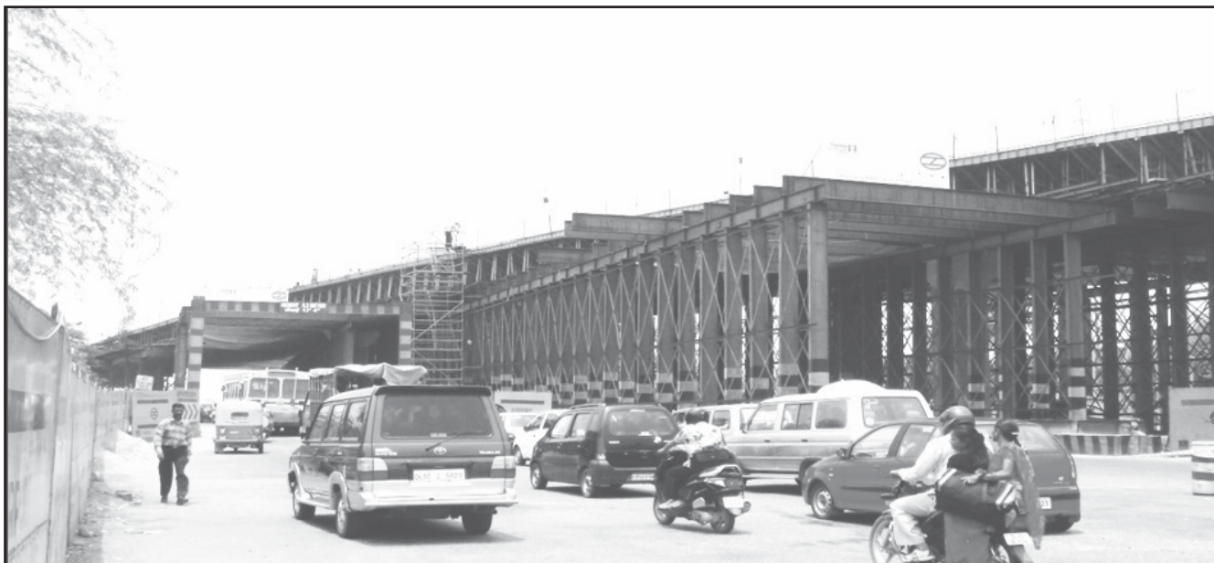
Figure 14. Temporary structure for casting continuous span at Dhaula Kuan
