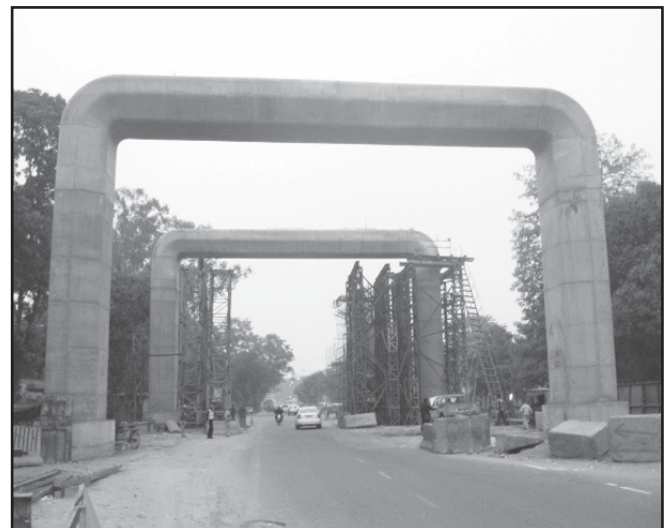
Figure 6. View of the highest portal pier, 16 m height
