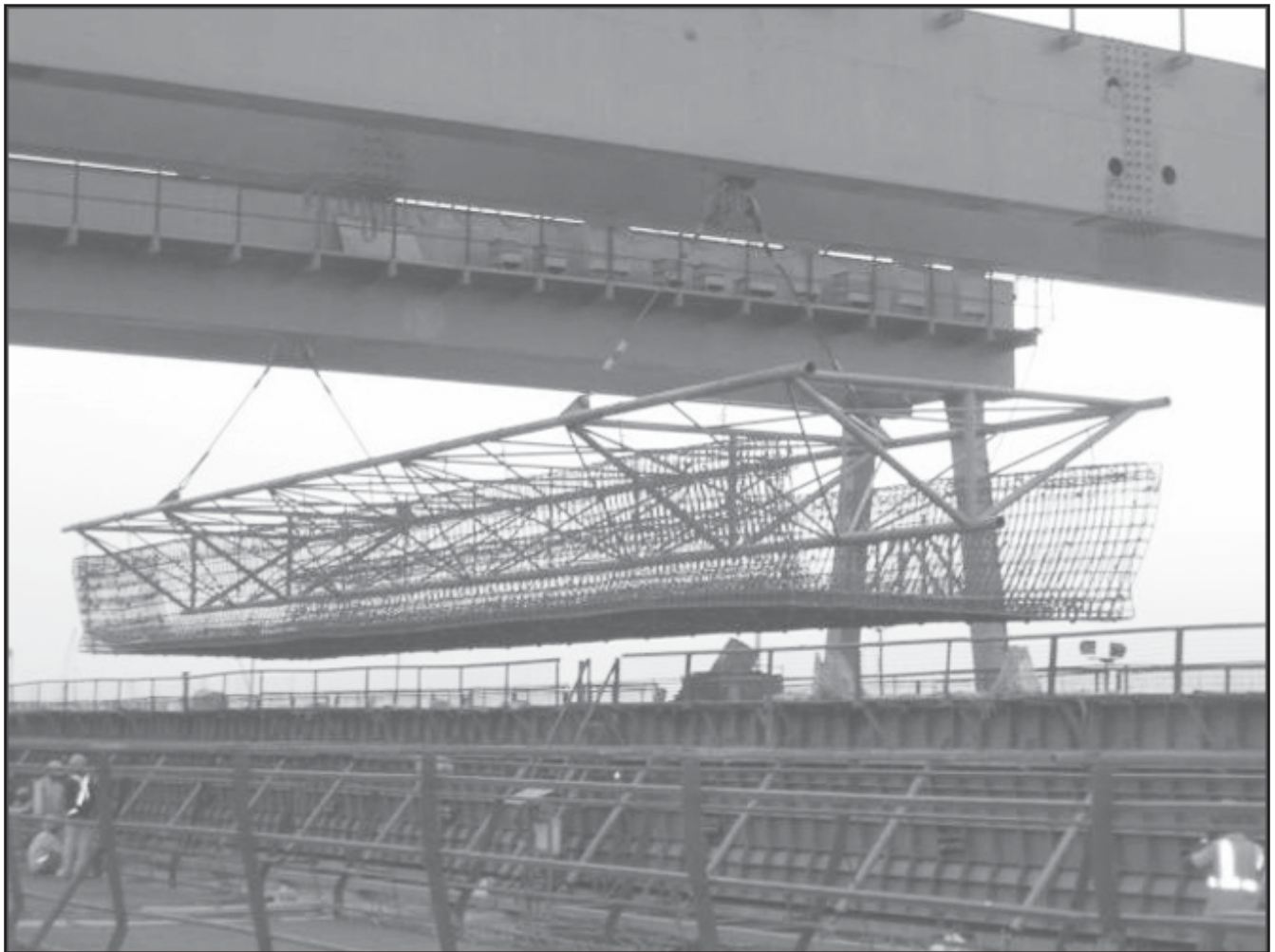
Figure 8. Placing of U girder re-bar cage
