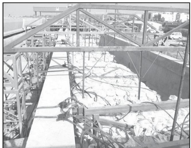
Figure 11. Load testing of the U girder
