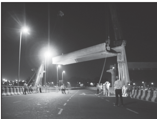
Figure 13. Erection of U girder at road flyover
