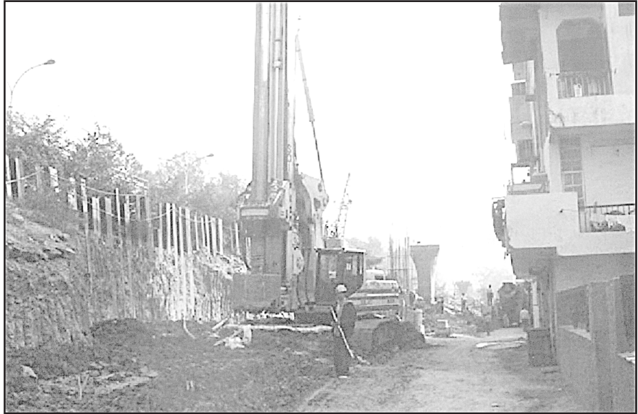
Figure 4. Piling work on slope of embankment
