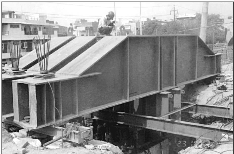
Figure 5. Pile testing being carried out
