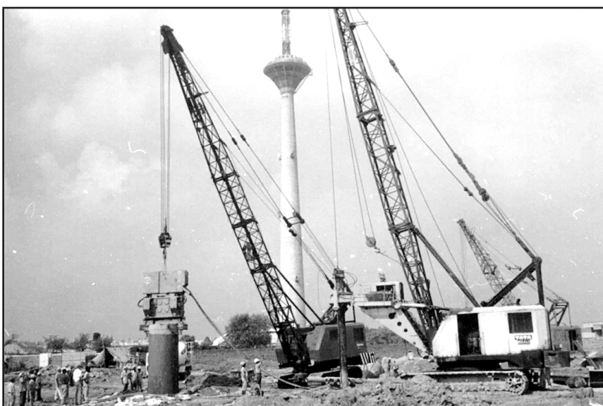
Figure 3. Piling work in progress
