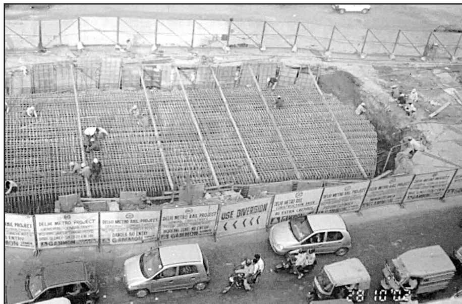
Figure 6. Reinforcement for pile cap laid in position
