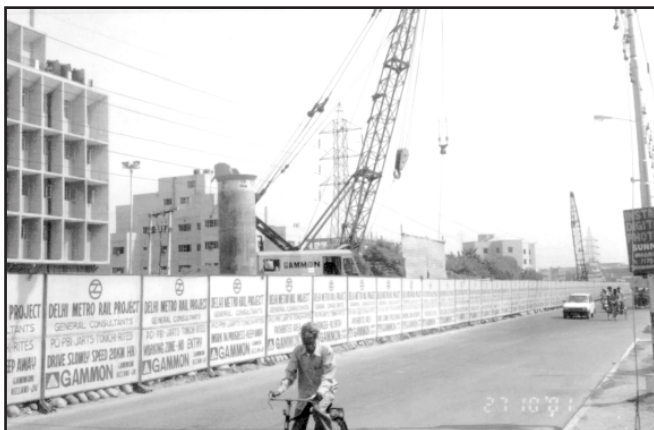
Figure 2. Barricade erected for separating construction activities from the road traffic
