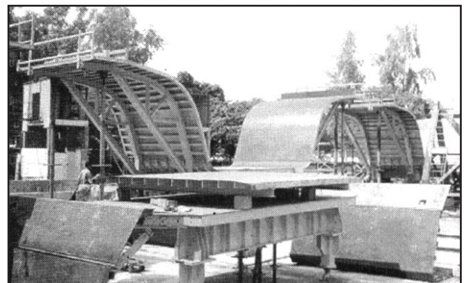
Figure 6. A view of the shortline mould
