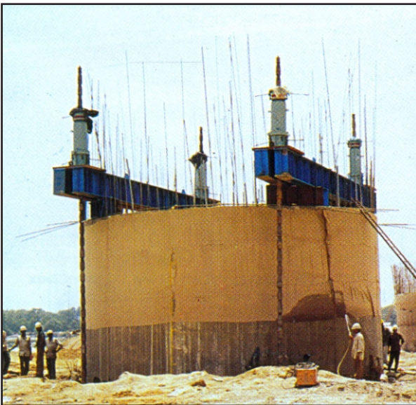
"Jack down" method of well sinking being employed
