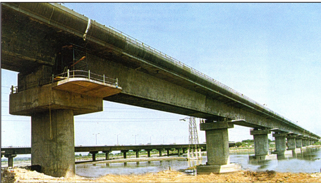
Last stages of superstructure launching is in progress as seen from rear end. Reaction was taken from concrete stopper over pier P14. Extended diaphragm at end of superstructure was connected to concrete stopper for launching purpose
