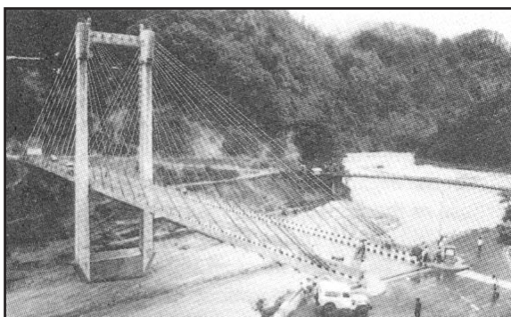
Figure 11. Akkar bridge in Sikkim — the first all-concrete, cable-stayed bridge in India.
