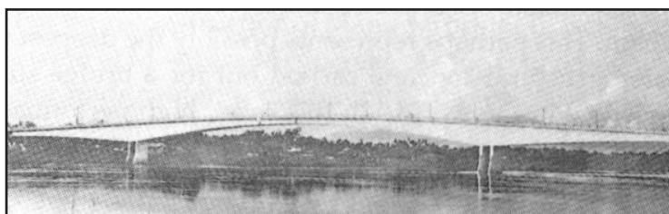
Figure 4. Barak bridge in Silchar, a long-span balanced cantilevered bridge with a clear central span of 122m.
