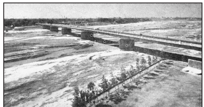
Figure 5. The Netaji Subhash Bridge at Ahmedabad is a balanced cantilever structure with main spans of 76.2m
