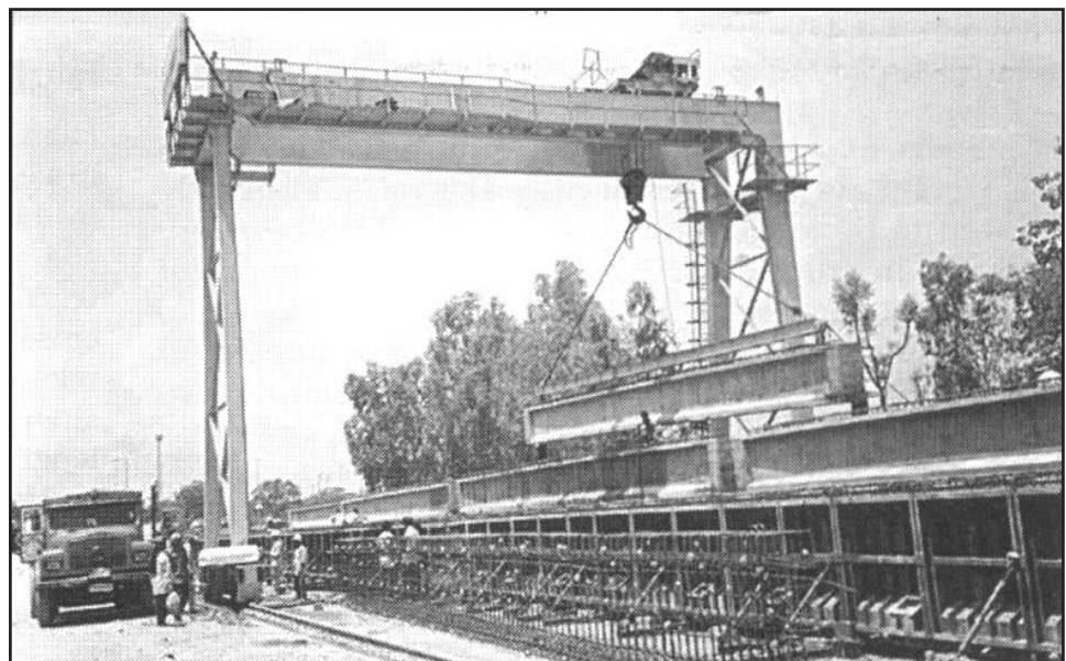
Figure 10. View of a typical precast pretensioned beam
