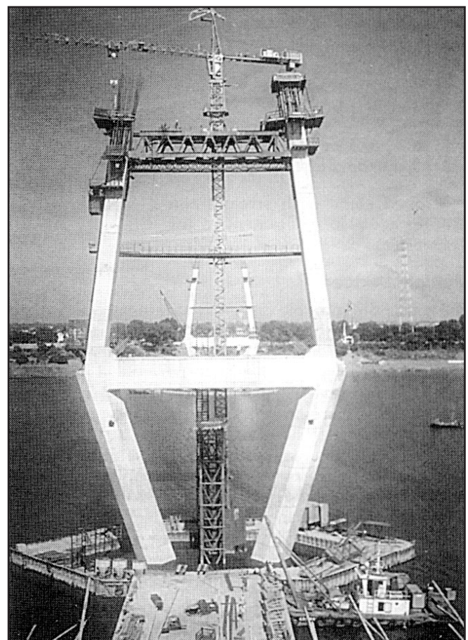
Figure 11. Pylon work in progress of the Yamuna bridge, Allahabad
