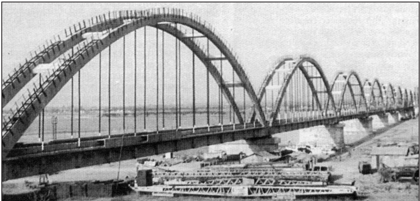
Figure 10. The third Godavari bridge, India (Source: BBR India Ltd. Bangalore)
