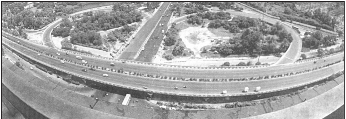
Figure 5. Clover Leaves at ITO Delhi: The sharply curved clover leaves connect the central artery (Vikas Marg) to the existing IP estate flyover
