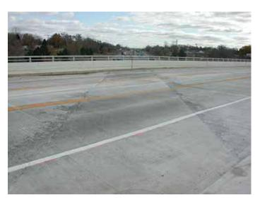
Figure 5: Condition of ECC link-slab immediately after construction and opening to traffic in 2005 and still in service in 2015. Apart from light abrasion on the surface of the link-slab, the condition remained about the same after 10 years of use.
