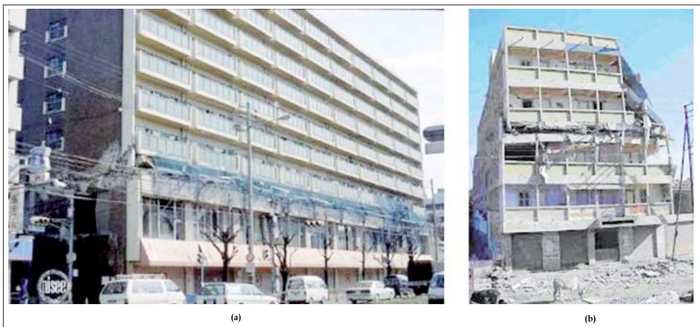
Figure 16. Examples of pan caking failure of buildings with soft storey at different levels
