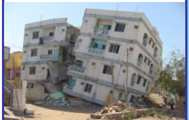
(b) Collapse of reinforced concrete columns (and building) during 2001 Bhuj (India) earthquake
