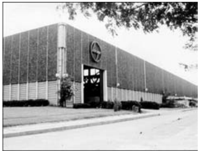
Figure 8. Larsen & Toubro Ltd., Bangalore - Hydraulic excavator project - 1975. Fixed concrete louvres in precast concrete wall panels
