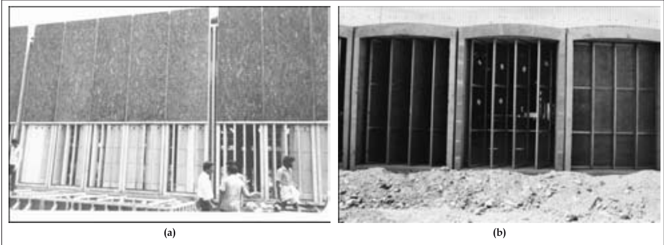
Figure 9. (a) A vertical rotating louvres of precast concrete at L&T, Bangalore (b) Vertical rotating louvres in galvanised iron with 'khus' for evaporative cooling - 1987
