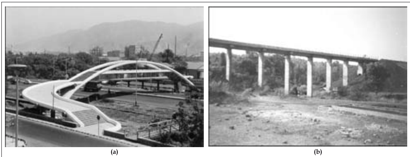
Figure 10. (a) Jainagar footbridge - 2002 (b) Berdewadi Nullah railway bridge
