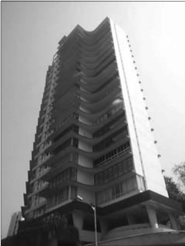
Figure 2. GESC apartment building - 1967
