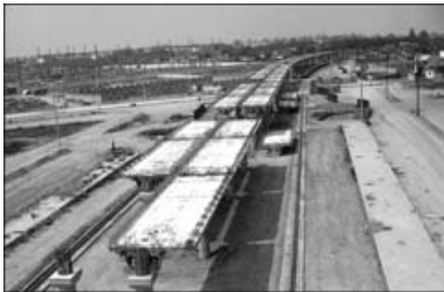
Figure 15. DMRCL 6.5 km long elevated viaduct - 2004
