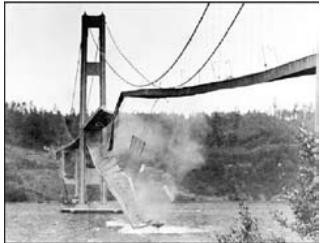
Figure 4. Tacoma Narrows bridge in Tacoma, Washington, 1940
