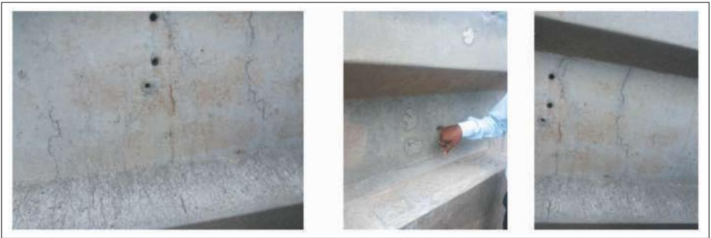
Figure 2. Cracks in girder
