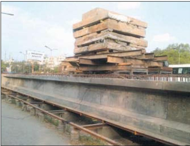
Figure 4. The loading arrangement during girder load test
