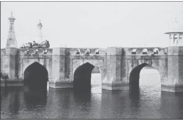
Figure 2. 'Sankh' Arch Bridge - Morena, Madhya Pradesh
