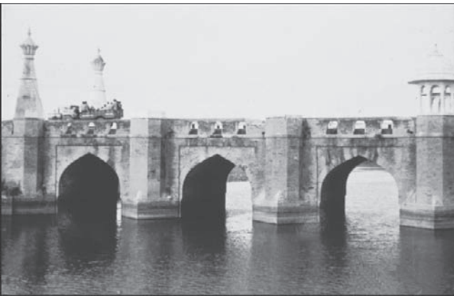
Figure 2. 'Sankh' Arch Bridge - Morena, Madhya Pradesh
