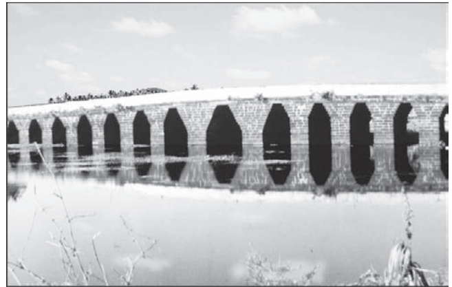
Figure 12. Corbel Bridge, Athar Nalla - Bhubaneswar (1000 years not out)
