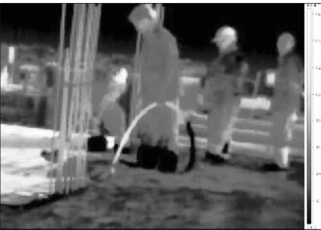
Figure 10. Hot weather concreting
