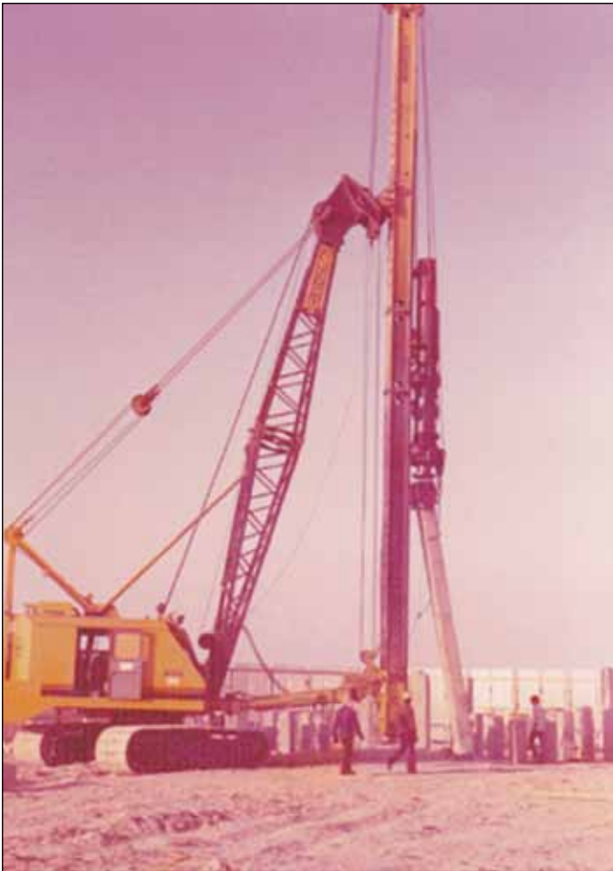
Figure 12. Precast prestressed concrete piles being driven at Abudhabi
