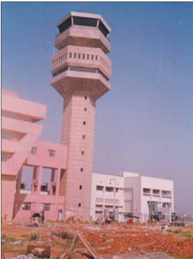
Figure 1. Control tower at Delhi Airport 55 m high (Year 1993)
