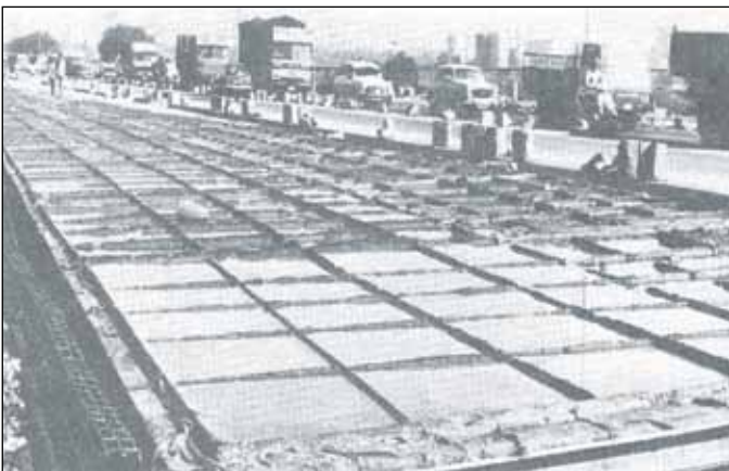
Figure 9. Ponding on a pavement slab for curing
