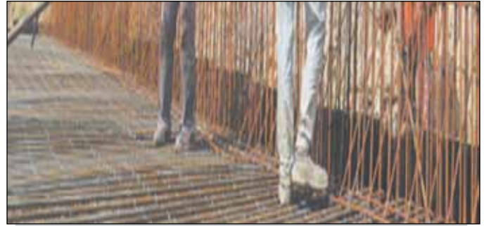
Figure 3. Reinforcements tied with knots placed in cover zone
