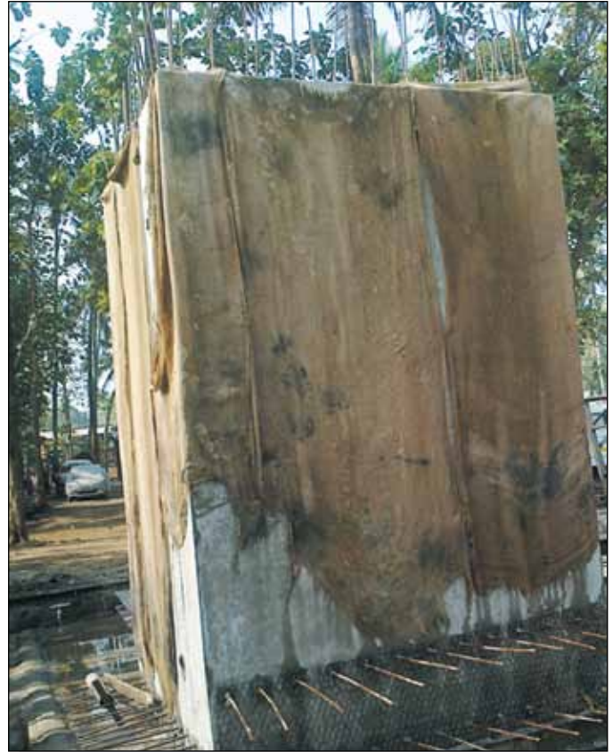
Figure 11. Proper curing of precast concrete culverts cast vertically in yard
