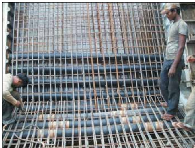
Figure 16. Fixing of HDPE sheathing for cables using inverted U-bars
