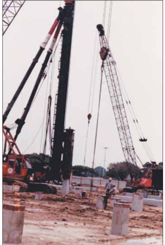
Figure 13. Precast RCC piles driven at a fertiliser project in India
