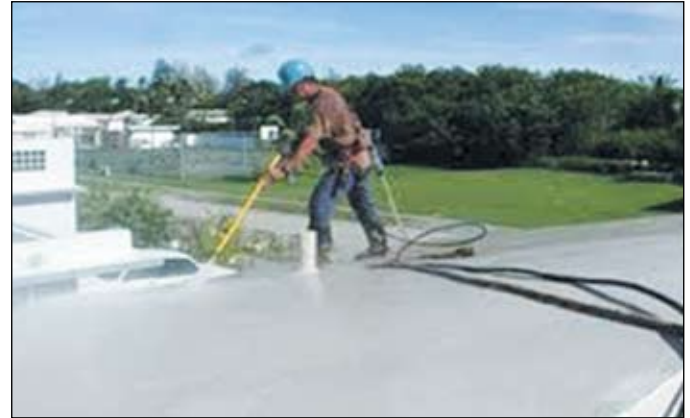
Figure 4. Membrane curing
