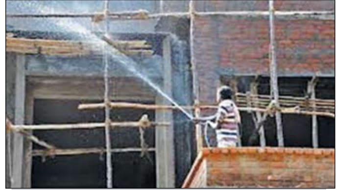
Figure 8. Water spraying curing method
