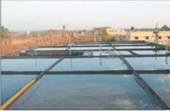
Figure 7. Water pond curing
