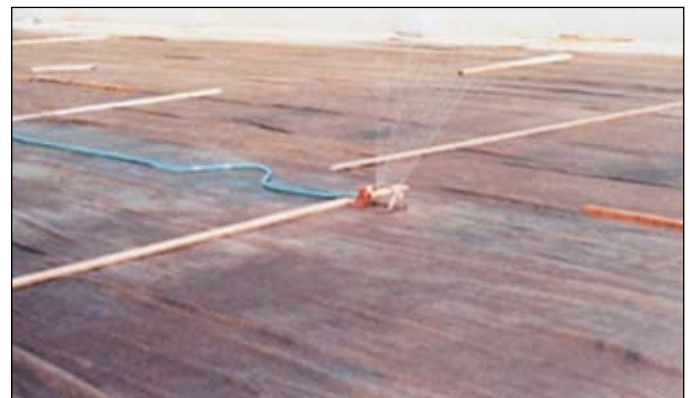
Figure 6. Curing using Jute bags covering
