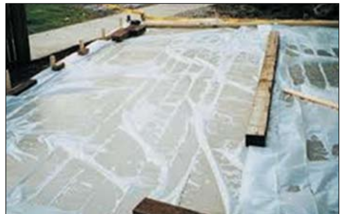
Figure 5. Curing using plastic sheet or tarpaulin
