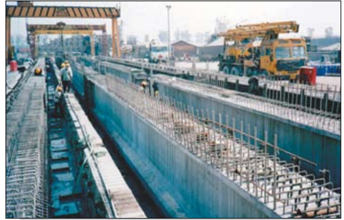
Figure 8. Curing water recirculation in manufacture of long pretensioned girders
