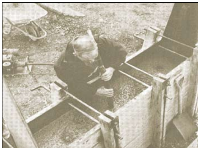
Figure 7. Poker vibrator in use [10]
