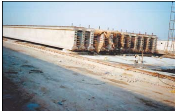
Figure 6. Precast pretensioned girders cast with steel formwork, stacked in yard
