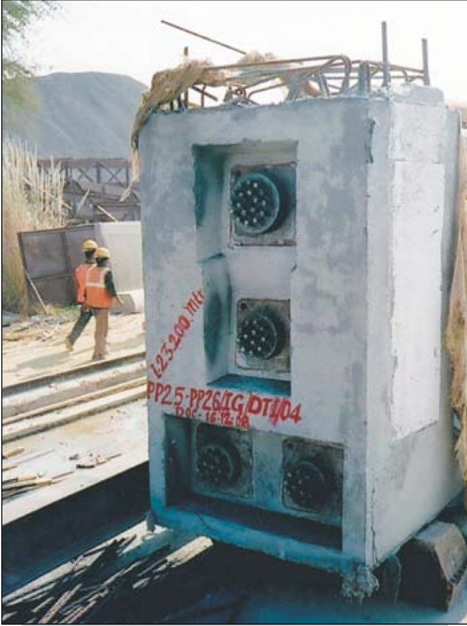
Figure 4. Good quality concrete in end block of a PSC girder
