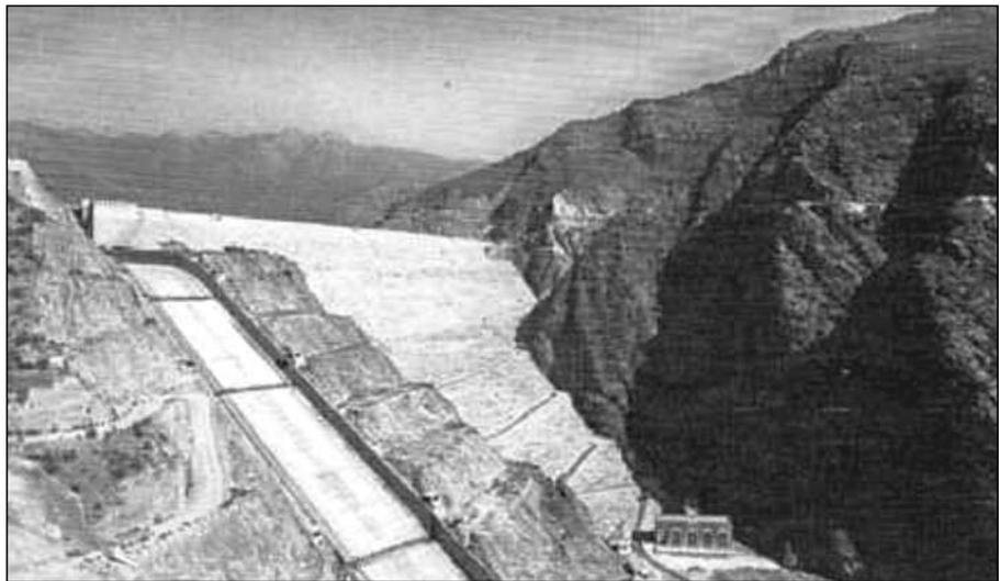
Figure 2. The spillway of 1000 MW Tehri hydro electric project uses 60 MPa concrete 8% silica fume
