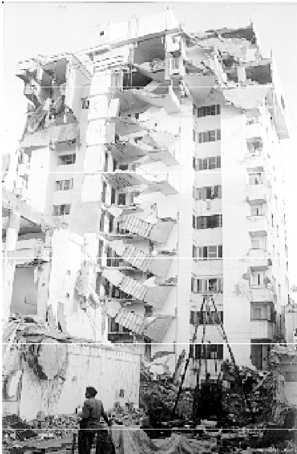
Collapse of a multi-storeyed building. Besides many reasons for failure, the main reason was additions and alterations done without considering earthquake forces
