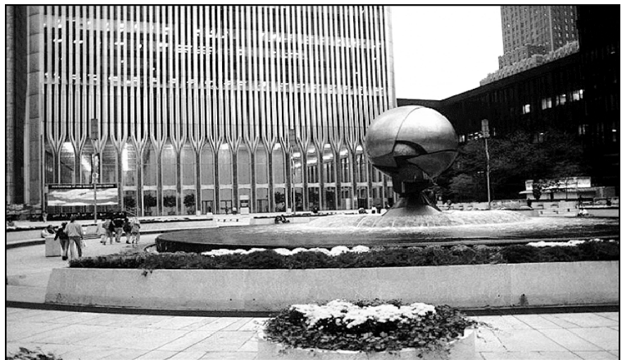
Fig 1 View of the entrance of World Trade Centre (Note the close spacing of columns)
