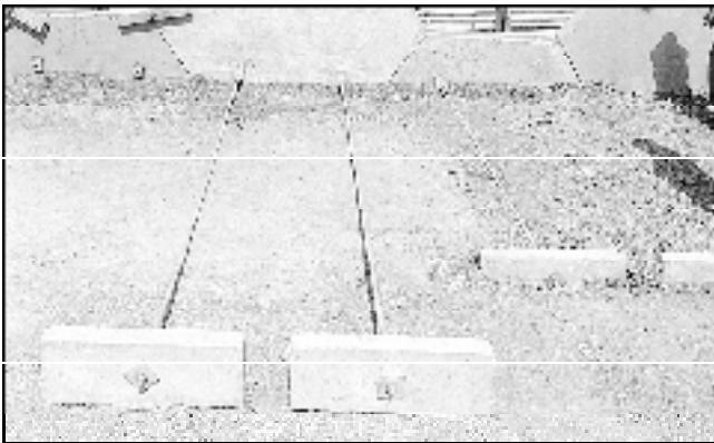
Fig 3 Anchored earth system with metallic bars and anchor blocks, licencees: MBN Anchored Earth Ltd
