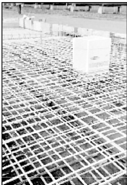
Rebar in concrete (structural pultruded elements)
