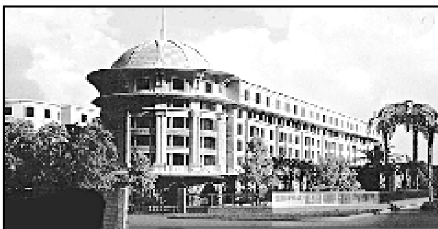
GRC Dome Cladding - ITC Grand Maratha Sheraton, Mumbai
