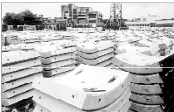
Glenium 51 is used for precast sections of tunnel works at Ghatkopar, Mumbai
