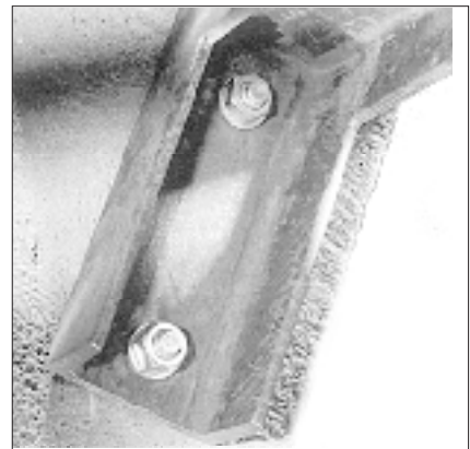
Installation example — fischer anchor bolt FAZ
