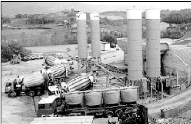
MEV batching plant in operation
