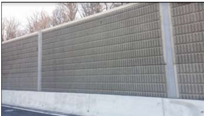
Figure 9. Noise barrier along a highway in Virginia, USA
