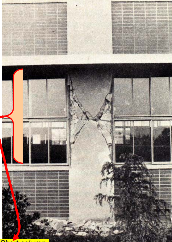
Short column between lintel and sill of window
